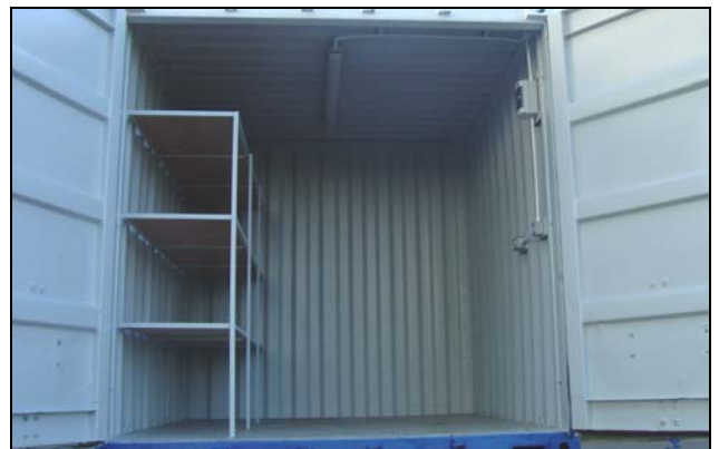
10' Cut Down - Electrics & Shelving
